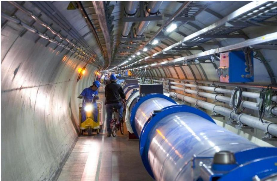
**Perspective of the LHC Tunnel: protons circulate in a beam pipe surrounded by superconducting magnets (in blue) used to bend their trajectory to a circumference.**
